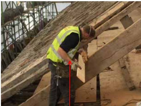
Joiner Andy making a template for a purlin repair
