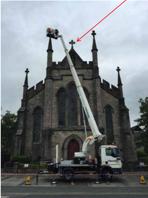
A footpath closure was required for the survey to be undertaken
