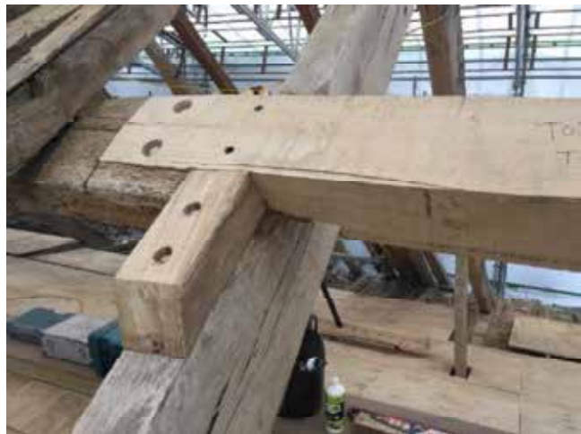
Completed purlin repair. Stainless steel fixings were used and a new oak block installed to give the purlin additional support
