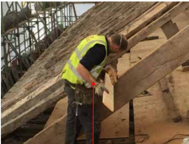
Joiner Andy making a template for a purlin repair
