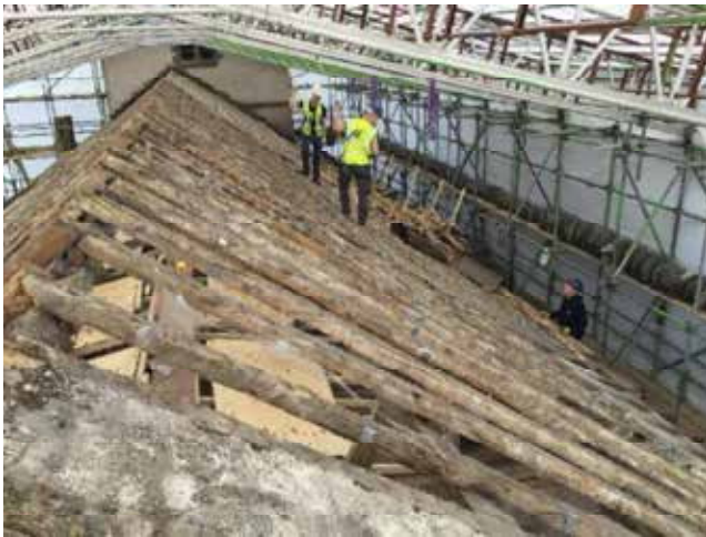
Slates being carefully removed and stacked in order, any replacement slates were slotted in at the appropriate place to ensure slates that were remaining went back in their original position
